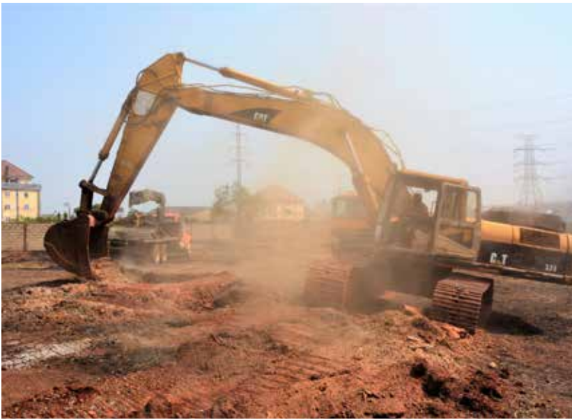
Digging the foundations ▲
